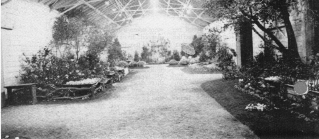
Building Number One
